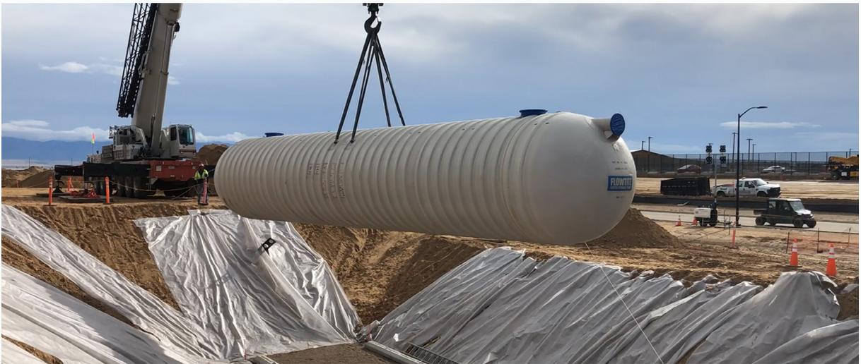
For our Los Lunas, New Mexico data center located in a desert climate, we engineered a system that captures rainwater from the roof in an underground cistern and cuts in half the amount of potable water needed to irrigate the surrounding campus landscape.
