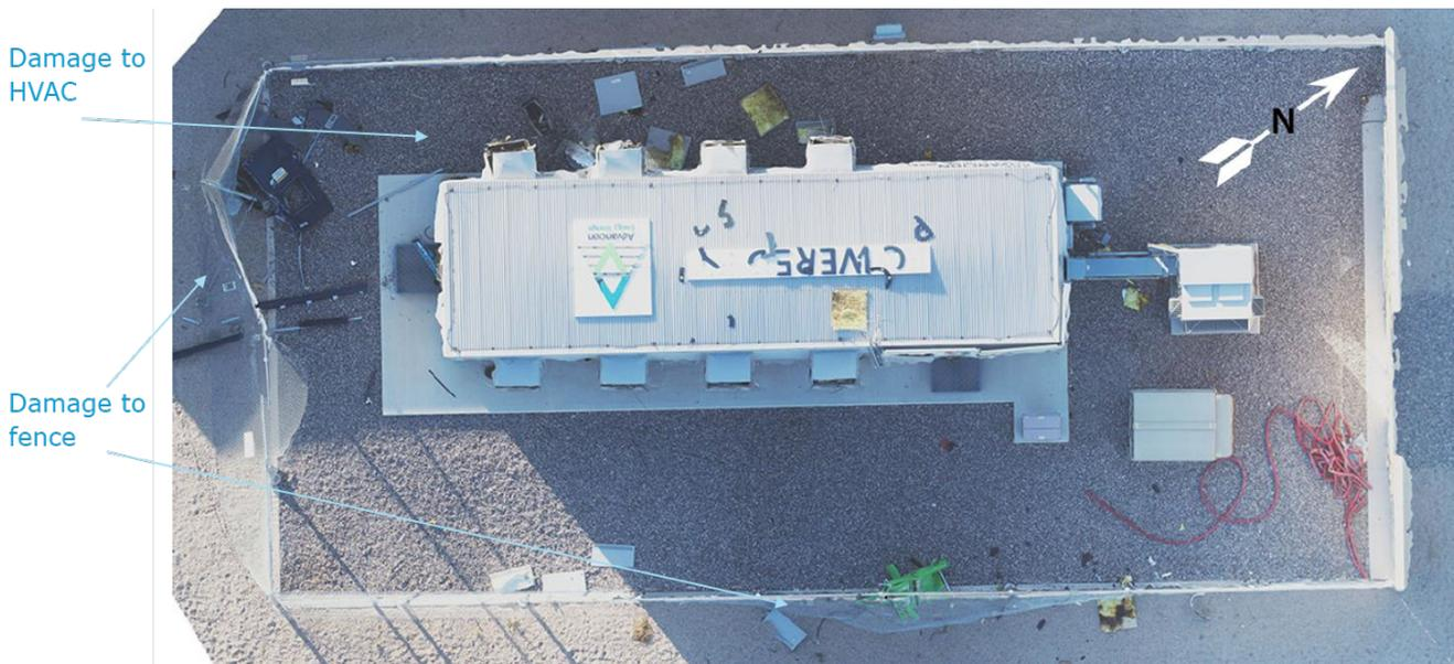
**Figure 5 Aerial view of damaged BESS (image credit: Colwell Consulting)**
